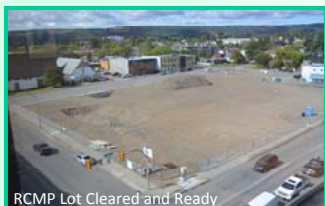
RCMP Lot Cleared and Ready
